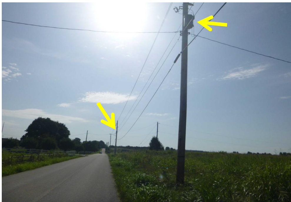
2. East - View of typical pole-mounted transformers (indicated by the arrows) located on the northern portion of the Site.
