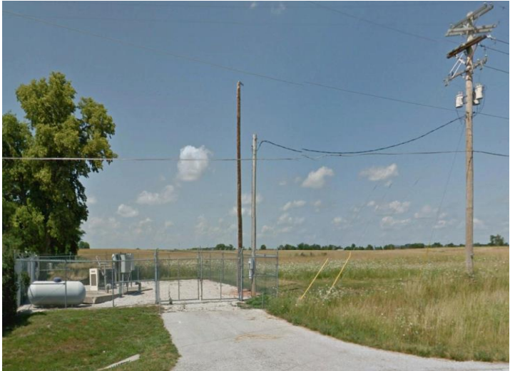
Photo #32 Lift station located at the southwest corner of the property. View of pole mounted transformer.
