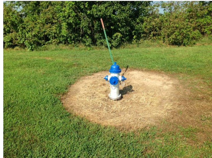
Photo #12 Representative picture of fire hydrants on site.
