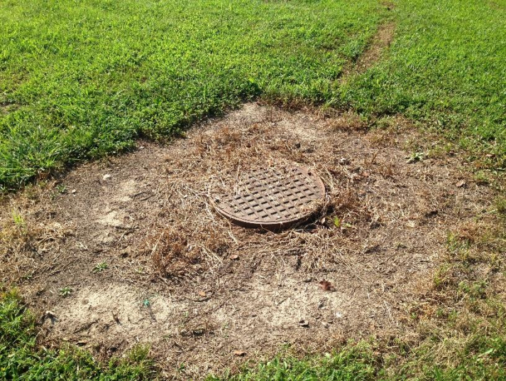
Photo #31 Sewer line manhole located at the northwest corner of the site.
