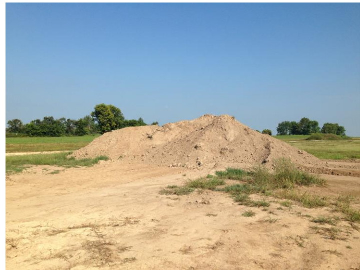
Photo #4 Dirt pile located in the center of the site.
