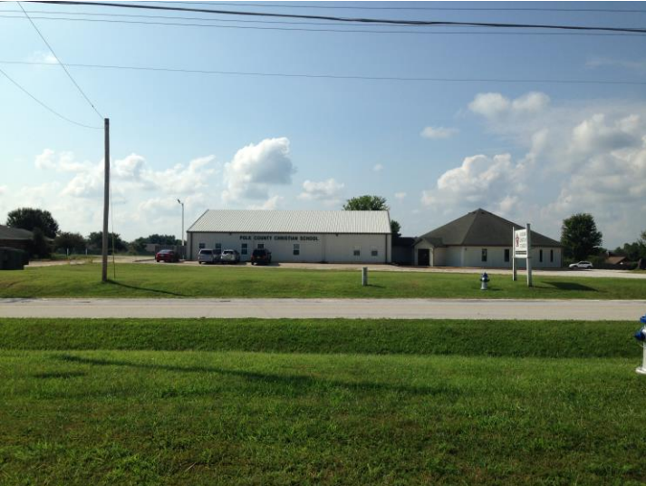
Photo #29 View of the south adjacent property across Tower Drive.
